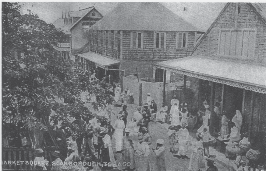
An early 1906 postcard of Market Square on Burnett Street. In 1816 all of the buildings were removed and it was declared that the Square be used for public purposes only.
